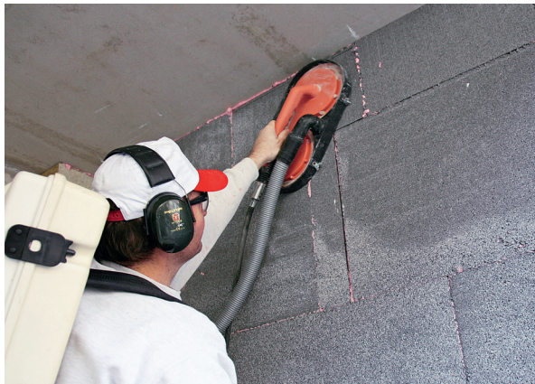
Grinding EIFS and ETICS boards
