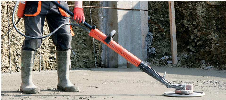
Levelling fresh concrete
