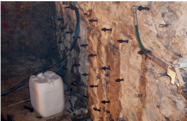
Positioning of packers on natural stone masonry
