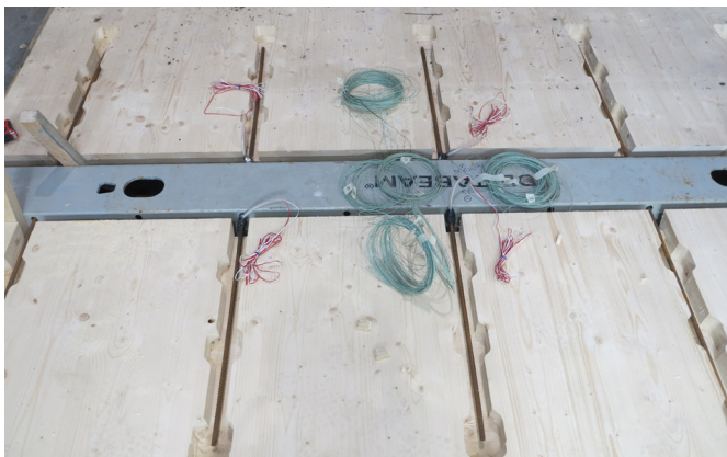
Figure 2. Transverse reinforcement secures the load transfer.
