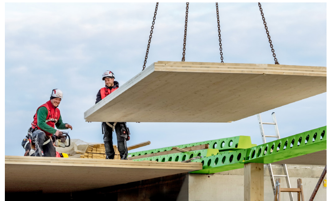
Figure 1. To increase sustainability Peikko's Slim Floor Structure solution is created with DELTABEAM® Green and CLT slabs [14].
