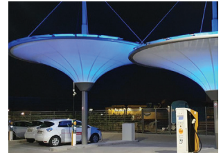
Energy station, Entega
