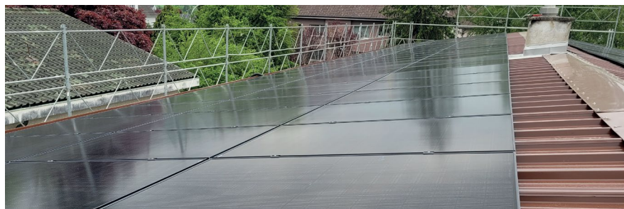
Roof renovation of a hall with the ROMA RD roof panel and integration of a PV system.
