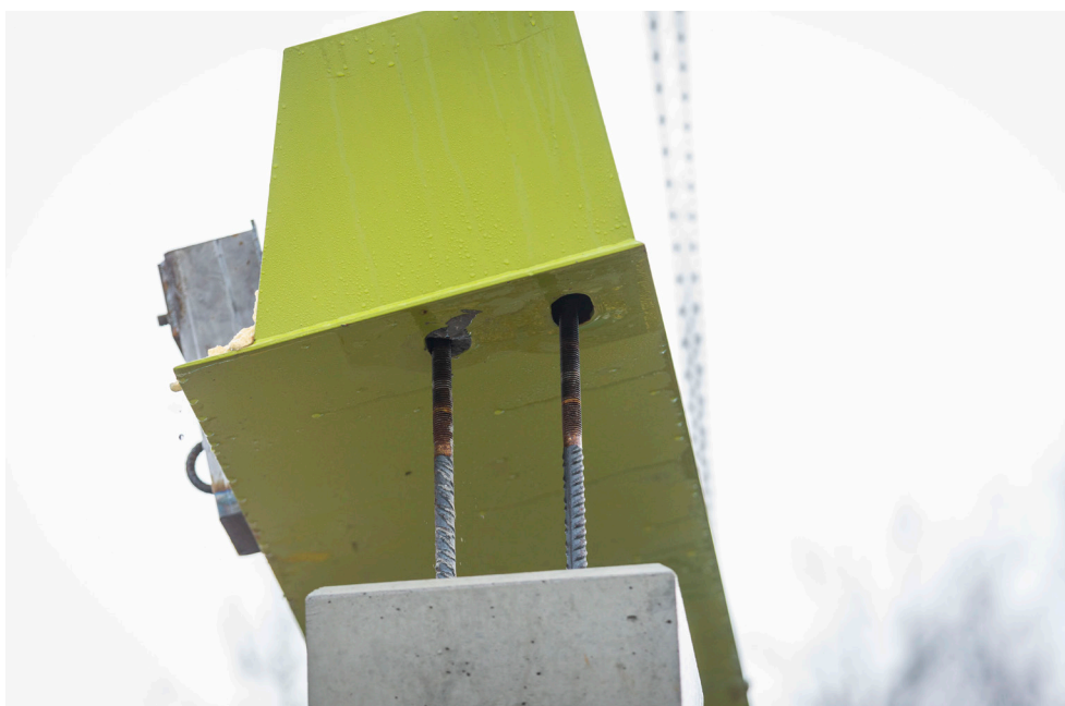
Figure 15. DELTABEAM® lifted off the column.
