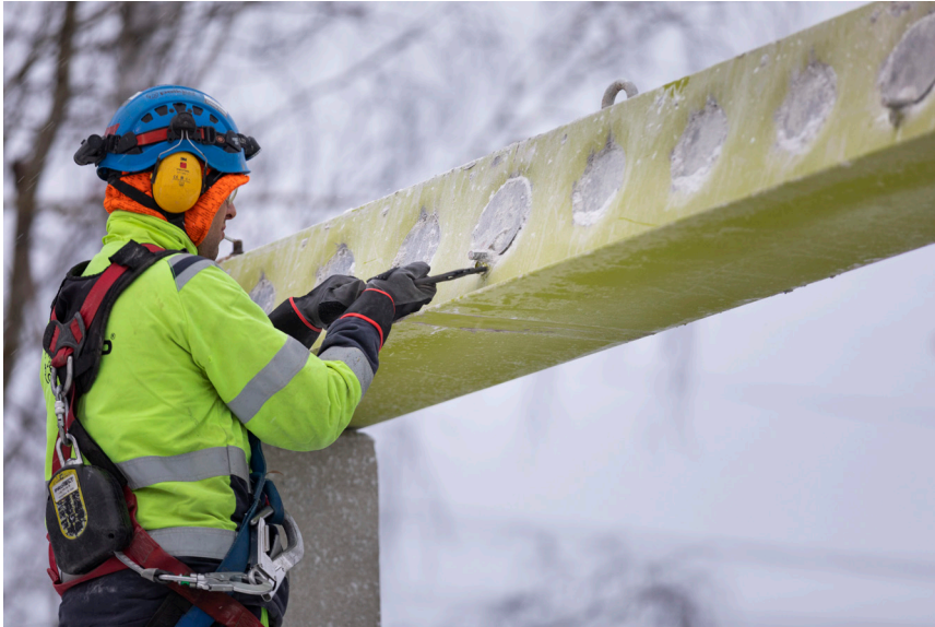
Figure 23. Removing of plug from MODIX® coupler A.
