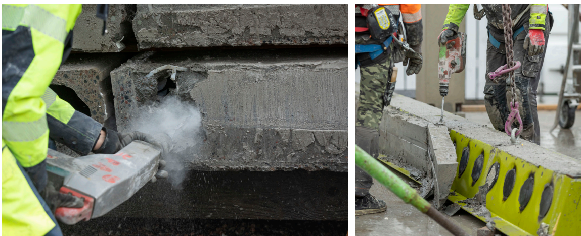
Figure 22. Cleaning of the elements (slab above and beam below) in preparation for reuse.
