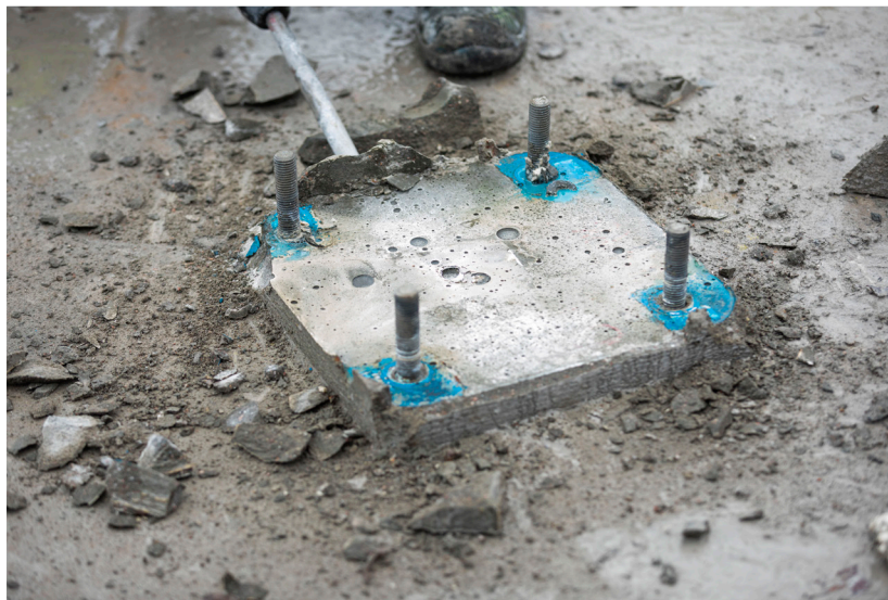
Figure 5. Removing of hardened grout pad.
