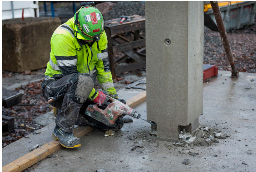
Figure 3. Removing of mortar off the recess boxes.
