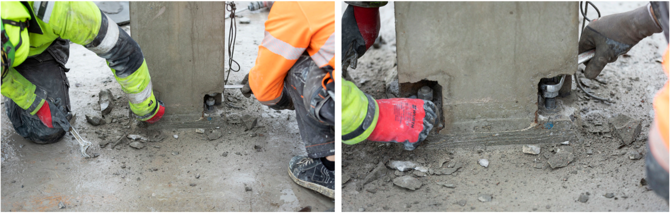
Figure 4. Opening and Removing of nuts.
