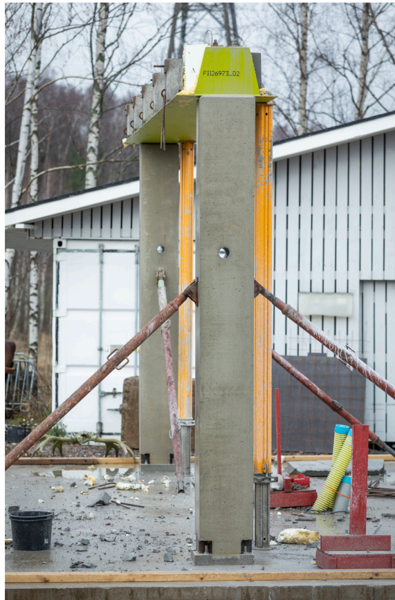
Figure 11. Supporting of beam using props, before dismantling.
