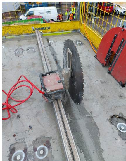
Figure 21. Diamond saw cutting through HCS longitudinal joints.
