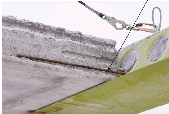
Figure 24. Part B of the MODIX® rebar coupler firmly screwed into Part A.
