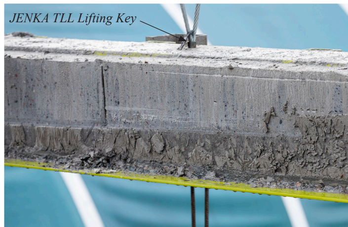
Figure 14. JENKA Lifting Key screwed into the DELTABEAM® Green, ready for lifting.
