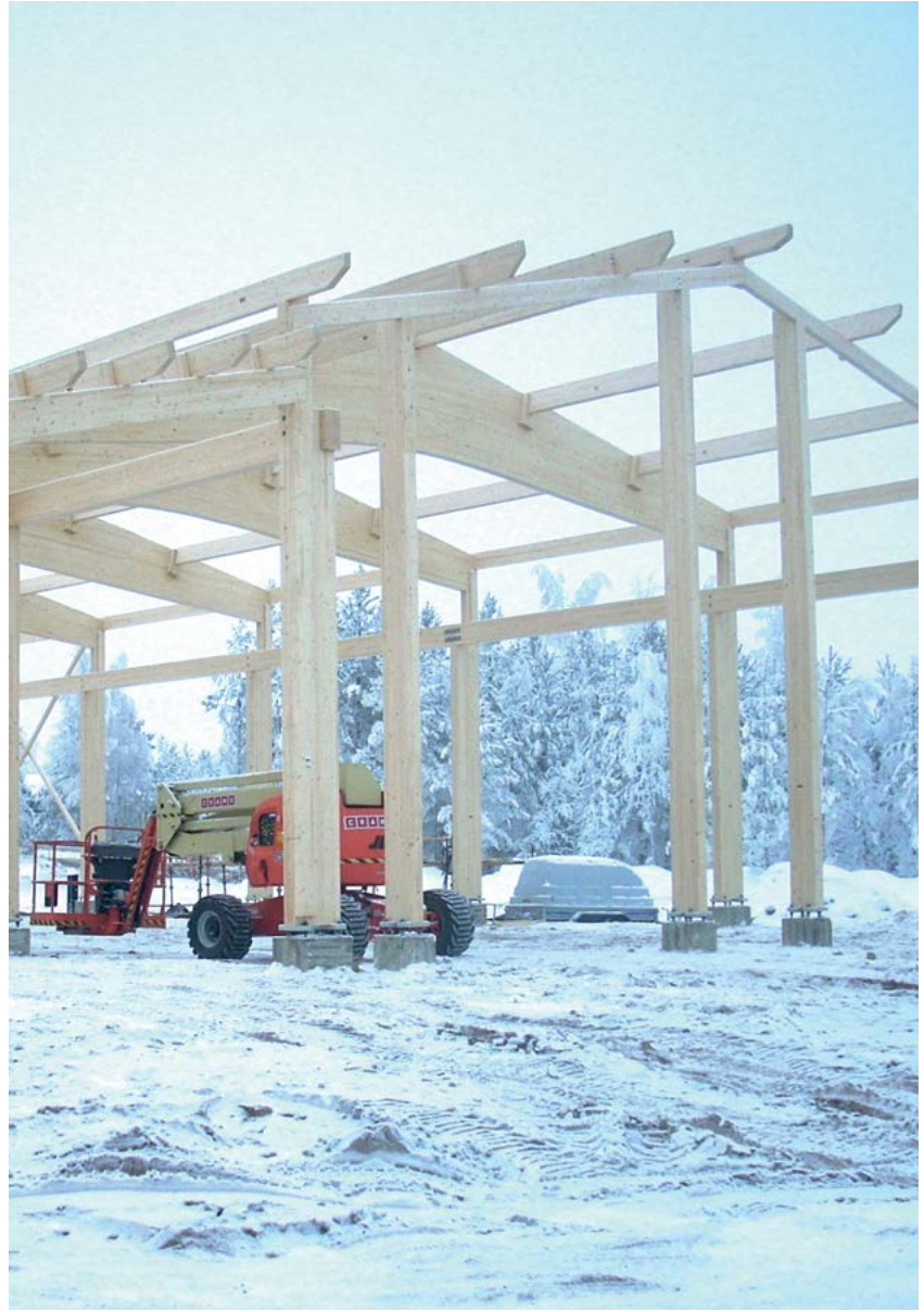
Industrial Hall, Valkeala
