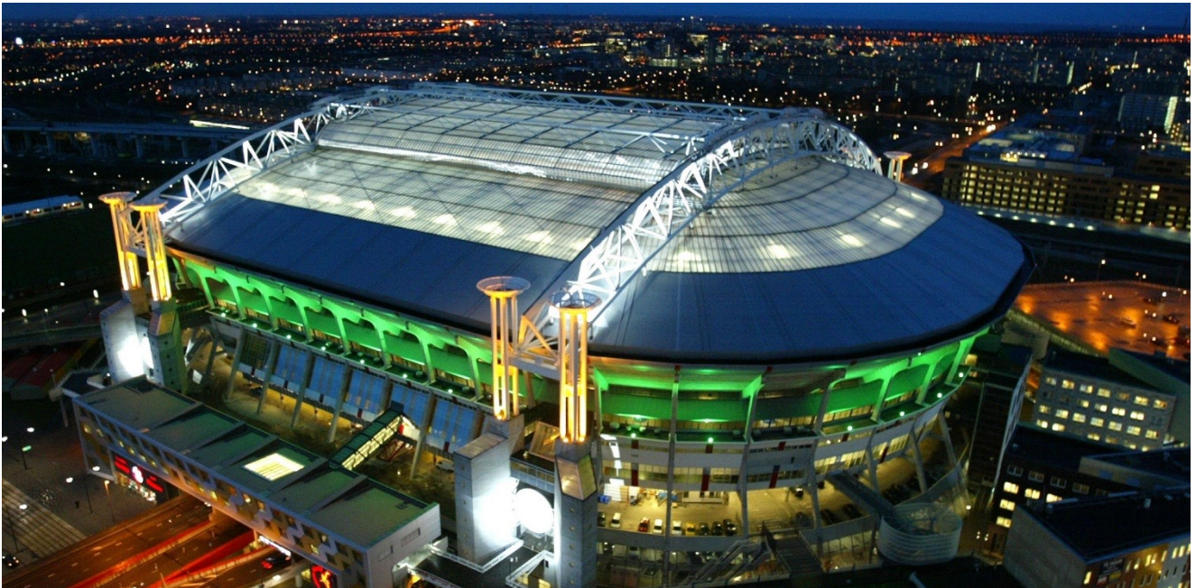
Johan Cruyff Arena, the Netherlands, LEXAN™ THERMOCLEAR™ Sheet has been in use since 1995, now 28 years!
