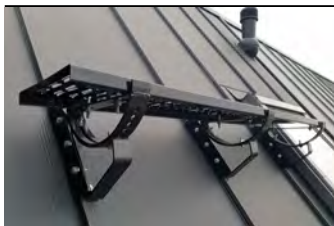
Steel roof communication for roof panels*
