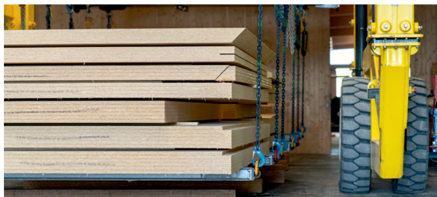
Loading of wall and ceiling elements
