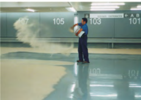
Quartz sand broadcast onto the fresh DUROFLOOR layer to reach the desired slip resistance in the Athens Concert Hall parking garage, Greece.
