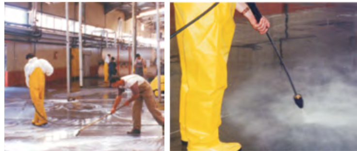
Hot water blasting to remove the oil from the floor.
