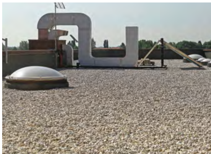
Gravel ballasted roofs
