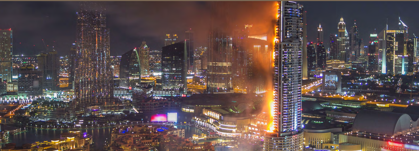
Fig.1 Fire event associated with combustible material on exterior cladding systems.
